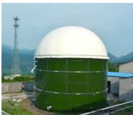
Figure 7: CSTR digester
